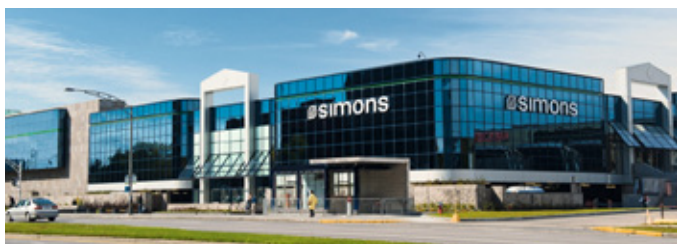
„Place Ste-Foy“ (Shopping-Center), Québec, Kanada
